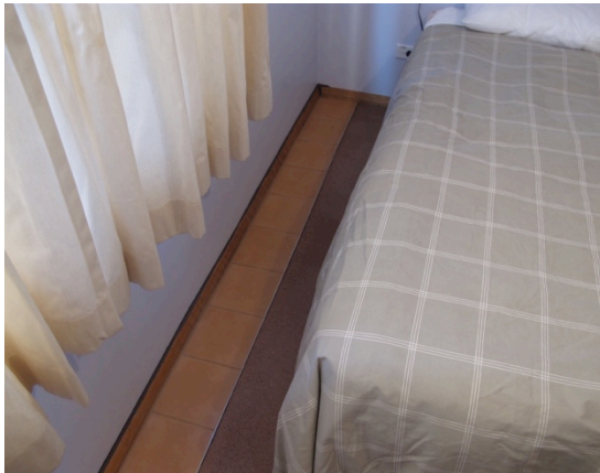
Waterproofing remedial work
