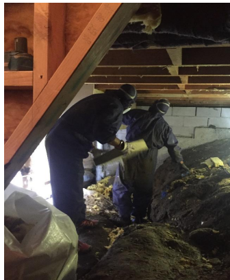
Installing New Insulation
