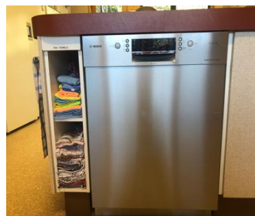
Four Dishwashers installed and featuring a tea towel Cubby Hole
