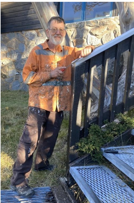
John repairing front steps
