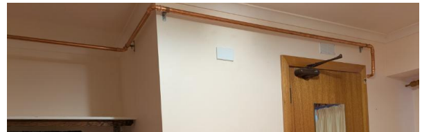
Sprinklers added to bathrooms.
