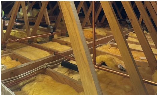
Ceiling space with foam lagging on some pipes.
